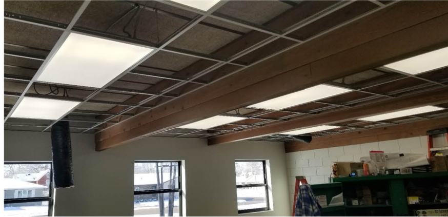
New classroom with ceiling grid and working LED lights!
